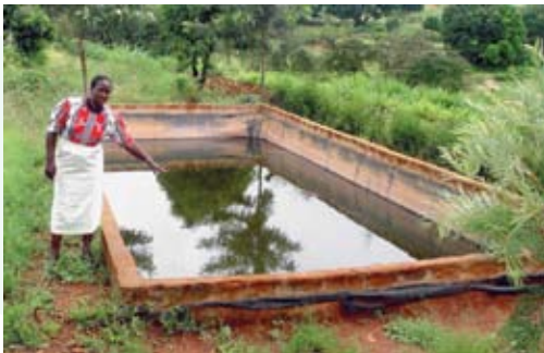
Plate 6: Farm ponds lined with ultra-violet-resistant plastic for micro-irrigation systems
