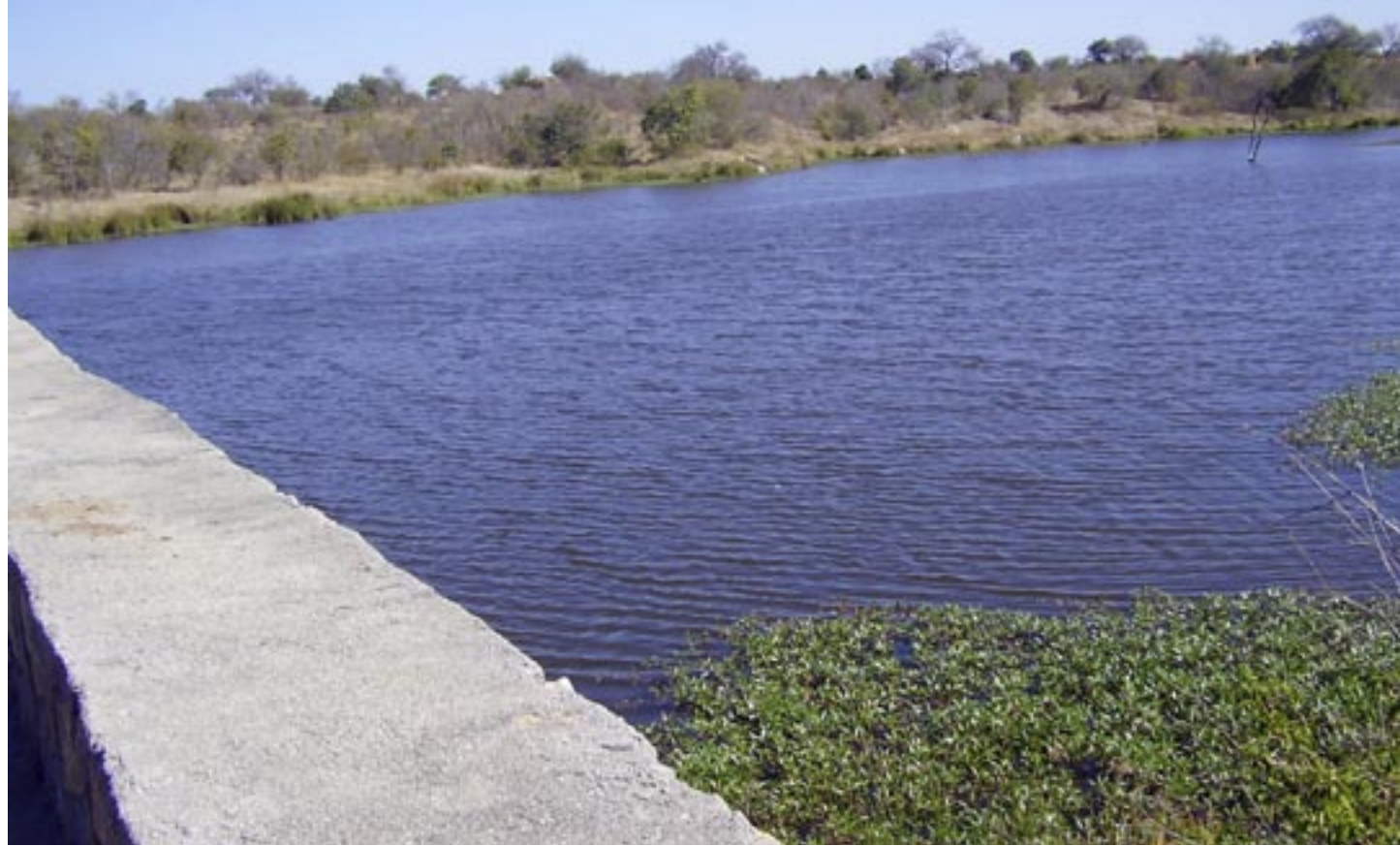
The recently built Nyiamai Dam enables communities to better manage the supply of water and irrigation of small farms
